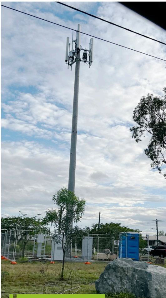
One of two new towers taking shape in Dysart.
